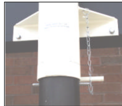
Figure 3-2 Safety Pin
